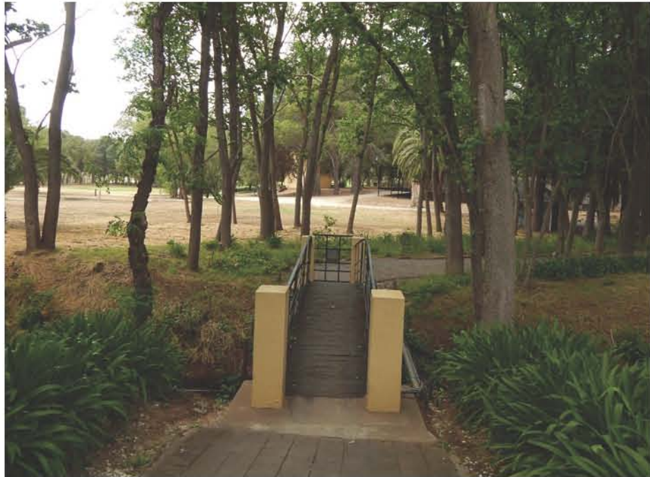
1 Elm walkway bridge
